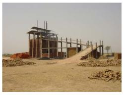
The unique feature in this VSBK is the construction of an elaborate L – shaped RCC ramp. This is not only used for green brick transportation to the loading platform but also as a store area for green bricks to be used for firing during rainy season.
