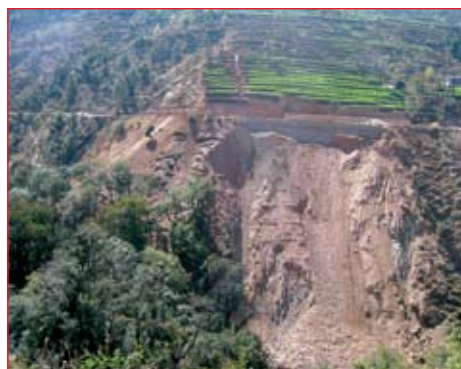
Land degradation – disturbed slope due to road construction (Bajang District)
