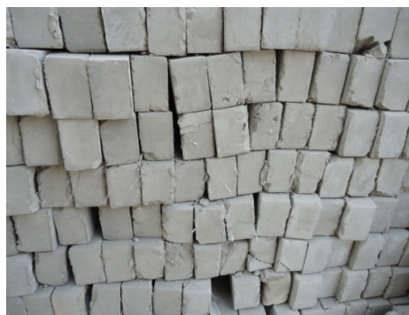
Figure 5: Poor quality of fly ash bricks a concern
