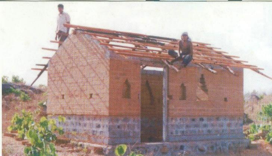
Left: Installation of roofing structure in local hardwood
