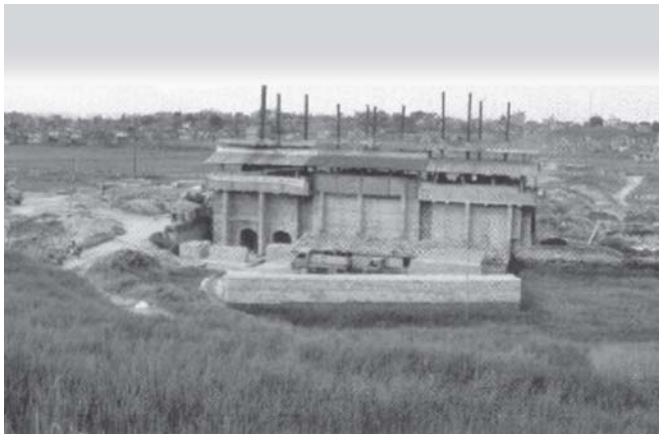
The pioneering 6-shaft VSBK near Kathmandu produces excellent bricks without pollution, all year round
