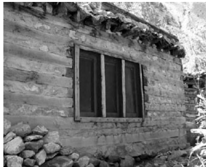
Stone masonry with timber bands in Rai Kot Valley, Gilgit survived the earthquake while all other stone masonry without such seismic features failed Source: schoolsafetyconference.org
