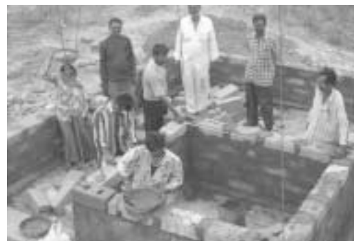
Mason Training of Concrete Block Wall
