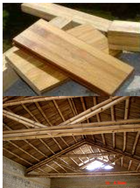
Figure 34: Bamboo Flooring Tiles (top), Bamboo Truss Roofing (bottom)
