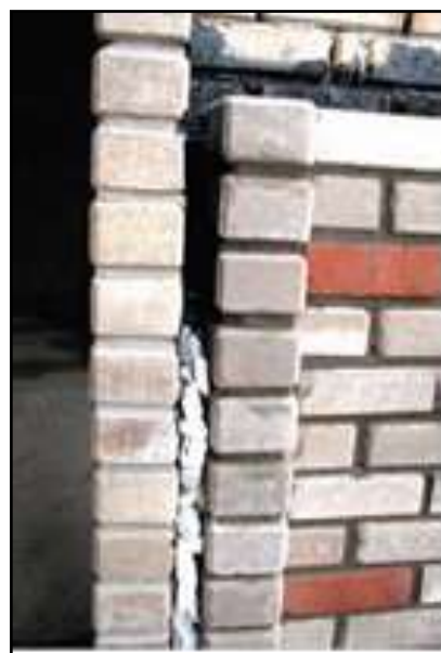
Figure 26: Cavity Wall with Waste Thermocol Infill
