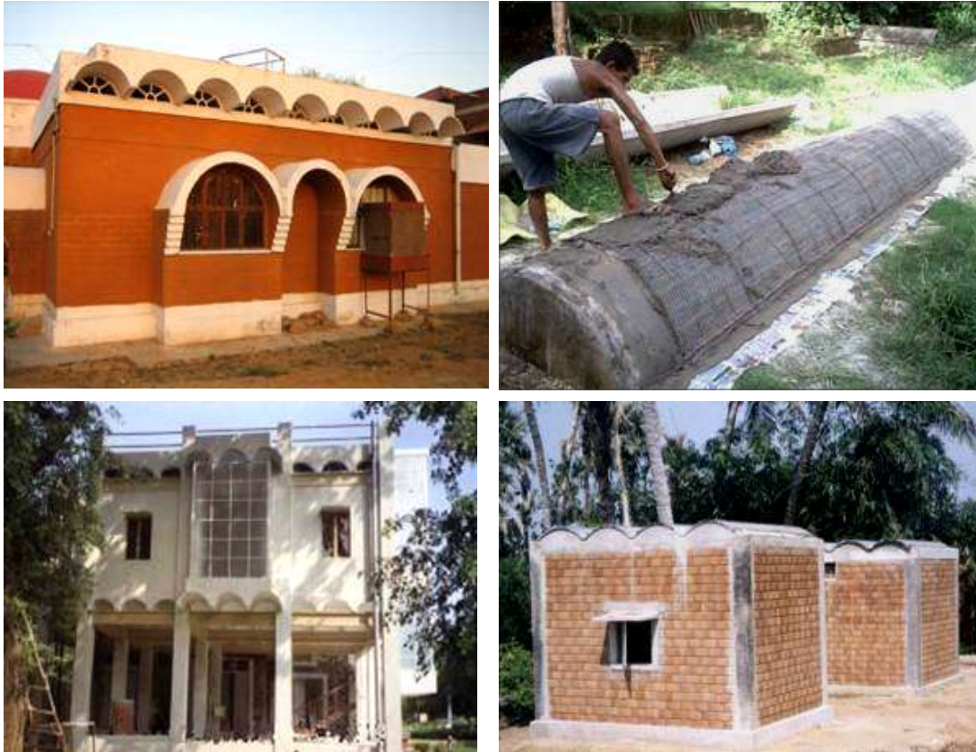
Figure 31: Ferrocement Channel Roof (clockwise from top left) Office Building in TARA Gram, Orchcha, Manual Production of Ferrocement Channel, Cyclone Resistant Shelter House in Orissa, Office Building in Delhi
