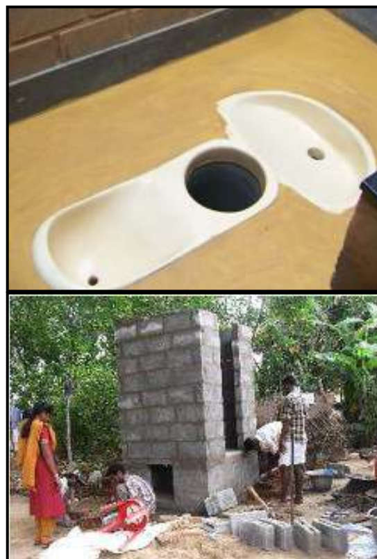
Figure 36: Ecosan Toilet on a Raised Platform with Waste Storage Below (top), Ecosan Pan for Waste Separation (bottom)
