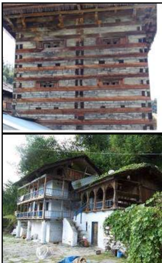
Figure 29: Wooden Logs as Ring Beams between Layers of Stone, External Verandas Resting on Massive Columns
