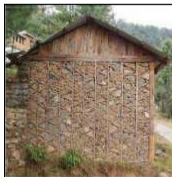
Figure 10: Traditional Dhajji Wall Construction in HP (top) and Stone Slate Roofing in Dharamsala (bottom)
