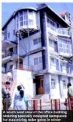
A south west view of the building showing sun spaces maximizing solar gains
