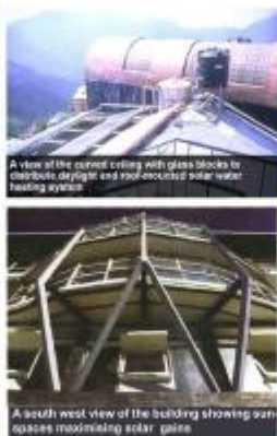
A south west view of the office building showing specially designed sunspaces for maximizing solar gains in winter
