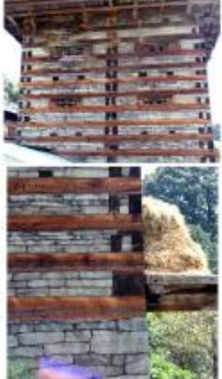
Elevation and corner views of timber reinforced stone masonry.
